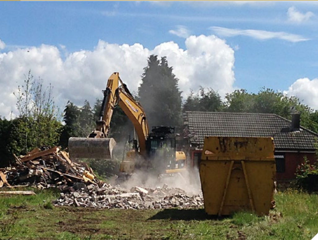
Demolition of Former Residential Property
