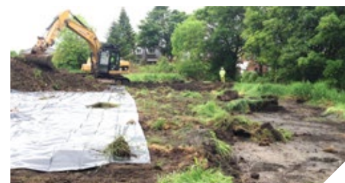
Himalyan Balsam Excavation
