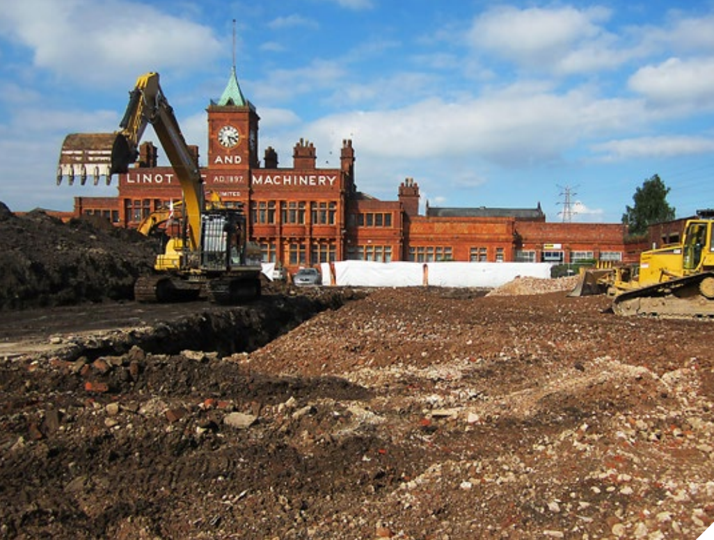
Controlled Excavation of Peat and Site Re-engineering
