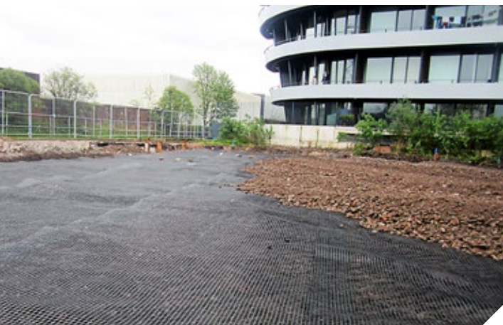
Geomembrane Installation to Bowling Green
